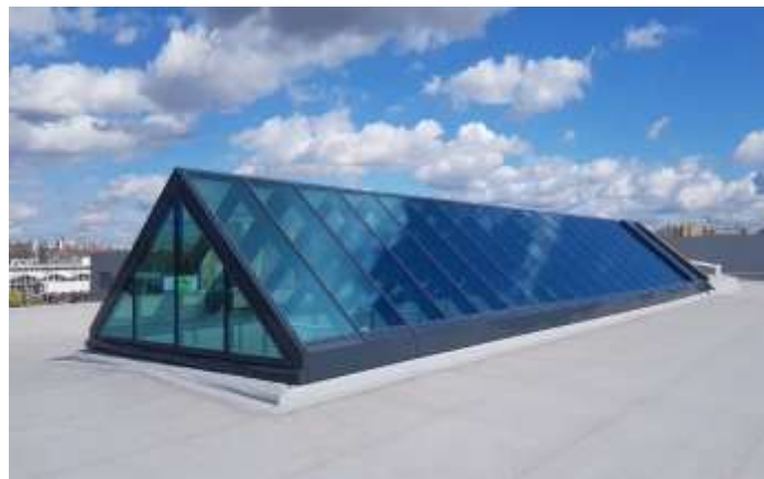
Figure 3: A high-slope glass roof that is not suitable for dust collection
