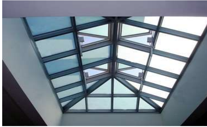
Figure 2: Low-slope glass roof suitable for dust collection
