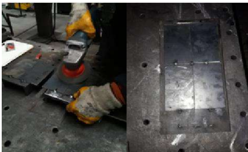
Figure 1. Surface cleaning process
